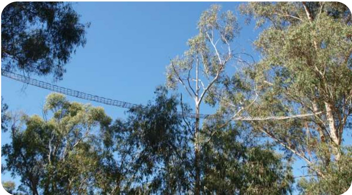
Figure 4. Wildlife canopy bridge on Wattletree Road, Eltham
