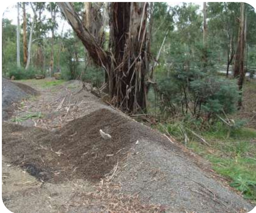
Figure 11. Excess materials should not be stockpiled against the base of a tree.
