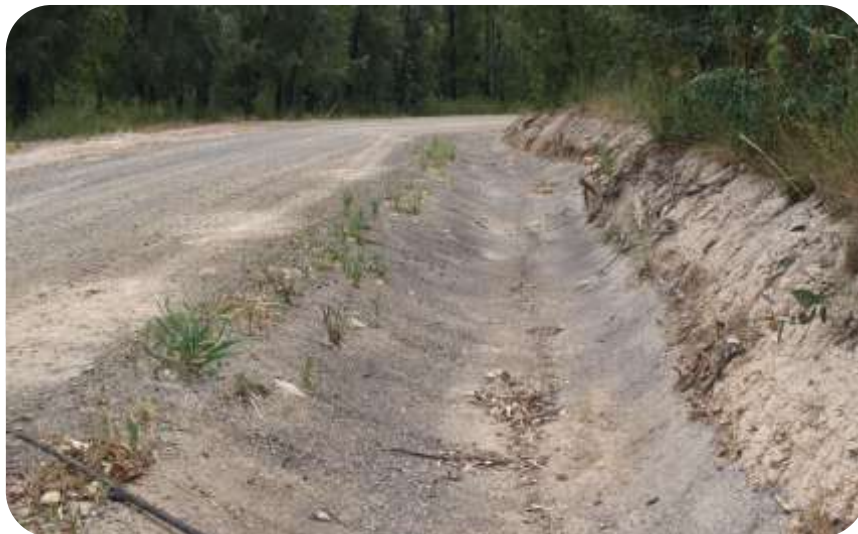
Figure 17. Cement-treated table drain on Rankines Road, Strathewen
