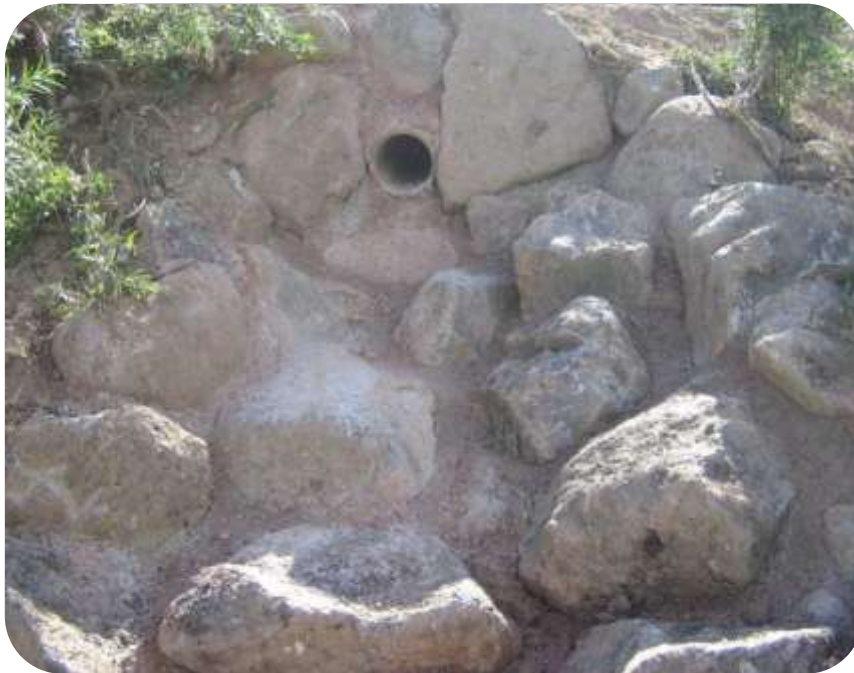
Figure 22. Rocking of culvert outlet absorbs the energy of run-off and traps sediment (Ninks Road, St Andrews)
