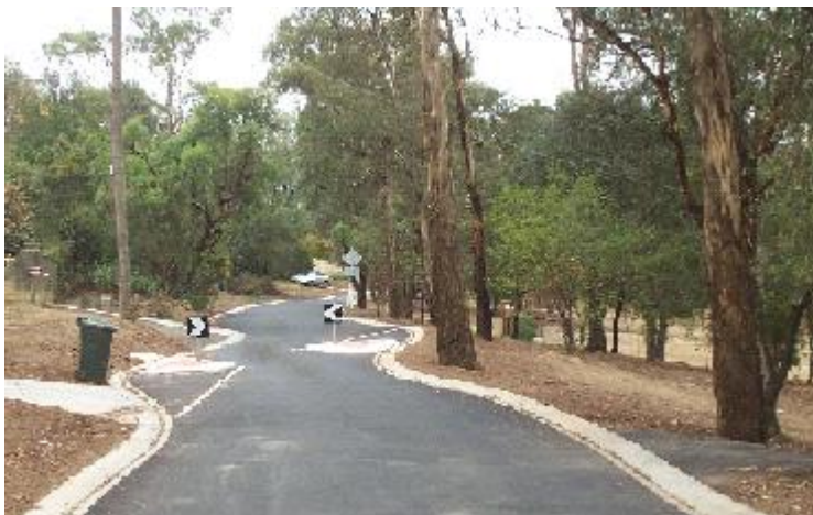
URBAN RESIDENTIAL ROAD CONSTRUCTION
