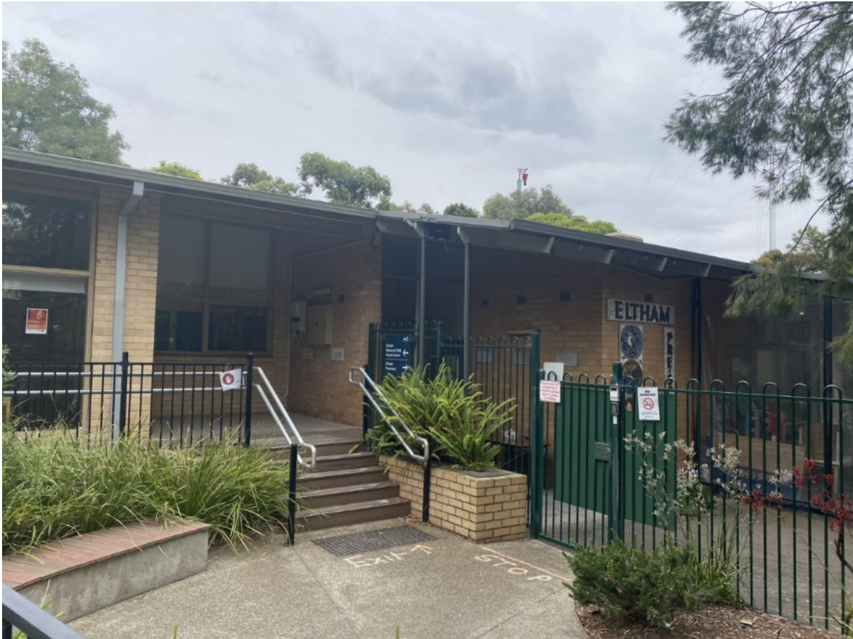
Figure 24. Principal elevation of the Eltham preschool. Entry to the preschool is through the recessed porch to the right of the planter. The entry to the left is to the former Children's Library added in 1961. (Source: Context December 2020)
