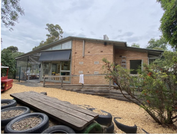
Figure 25. North elevation of the preschool building showing window wall, low-pitched gable roof and stepping in of building. (Source: Context, December 2020)
