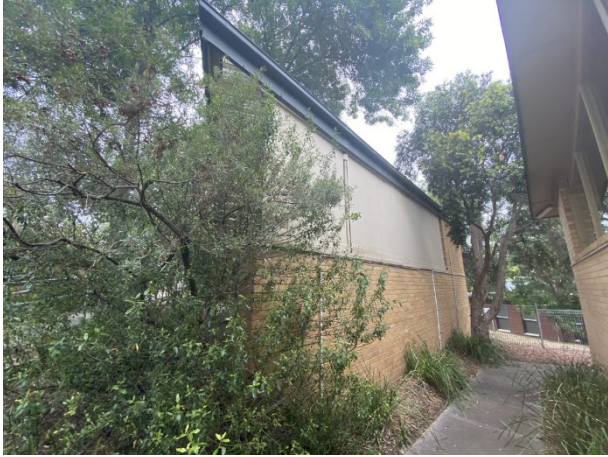
Figure 19. North elevation of the former Infant Welfare Centre showing dwarf closed wall above that was originally a louvered screen to pram porch. (Source: Context, December 2020)
