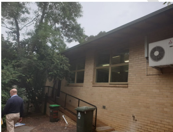
Figure 32. West elevation of War Memorial Hall (Source: Context 2020)
