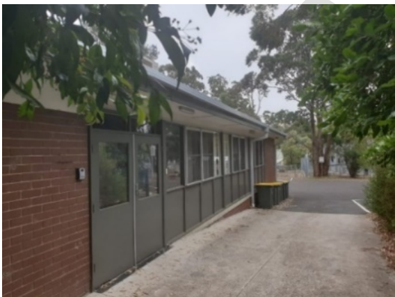
Figure 37. North elevation Senior Citizens Centre showing enclosed verandah with timber framed glazed wall. (Source: Context December 2020)
