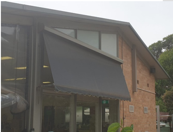
Figure 27. North elevation detail showing the top section of the window wall frosted as a false ceiling has been installed internally. (Source: Context, December 2020)
