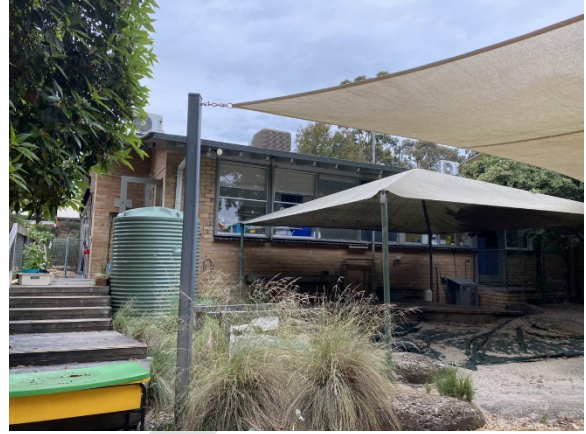
Figure 26. West elevation of the preschool building showing strip natural aluminium window with manganese brick sill. (Source: Context, December 2020)
