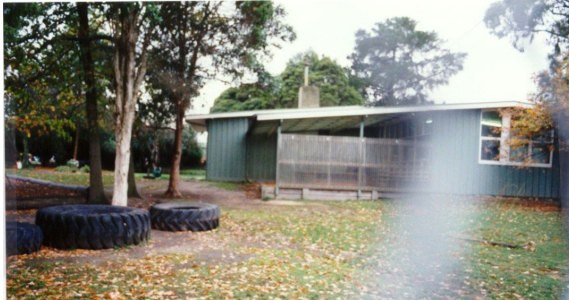
Figure 47. Greenwood Park Kindergarten, 9 Greenwood Avenue, Ringwood, built 1954-55 (HO28). (Source: Hermes)
