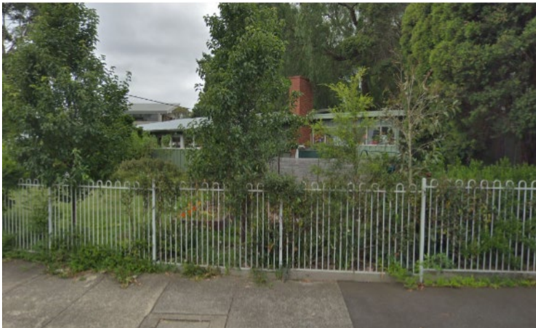
Figure 50. Armadale Memorial Kindergarten, William Street, Armadale, built 1951 (not in HO). (Source: Hermes)
