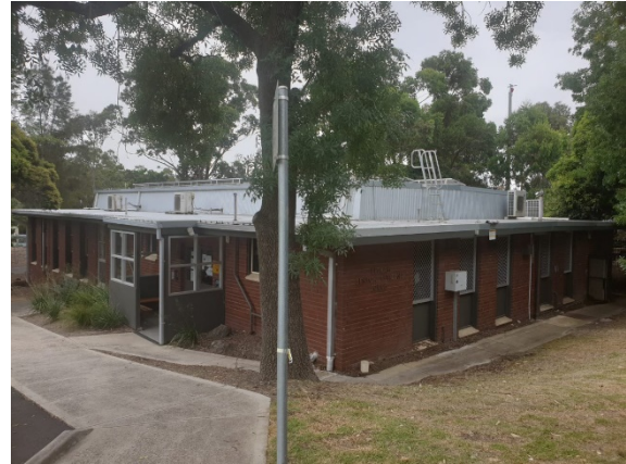
Figure 36. East elevation of the Senior Citizens Centre showing recessed window module with stone sill. (Source: Context December 2020)
