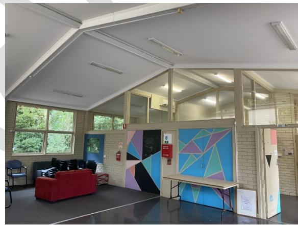
Figure 33. Interior of War Memorial Hall showing extant glazed partitioning system and expressed structural steel portal frame. (Source: Context, December 2020)
