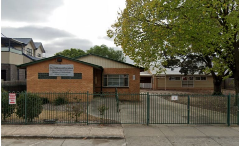
Figure 51. Glenroy Memorial Kindergarten, Glenroy (not in HO). (Source: Hermes)
