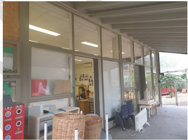
Figure 28. Window wall under verandah. Note the original eave overhand has been extended to create a deep undercover play area. (Source: Context, December 2020).
