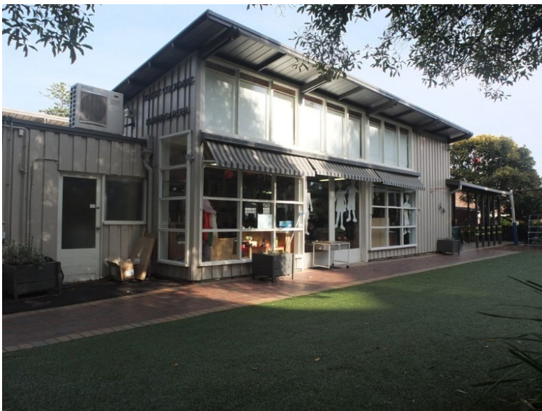
Figure 46. Robert Cochrane Kindergarten, 2A Minona Street, Hawthorn, built 1948-50 (VHR H2309, HO580). (Source: Hermes)
