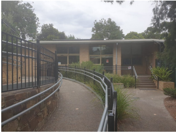
Figure 30. Principal elevation of Wall Memorial Hall showing ramped entry installed in 2012. (Source: Context, December 2020)
