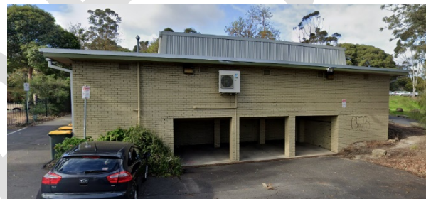
Figure 38. West elevation Senior Citizens Centre showing open basement car parking under the building. Note face brick work has been overpainted. (Source: Google August 2019)
