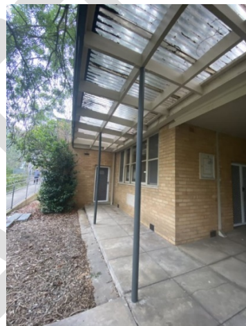
Figure 18. Pergola across principal elevation of the former Eltham Infant Welfare Centre showing slender metal posts. (Source: Context, December 2020)
