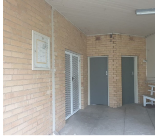
Figure 20. Pram porch at the former Eltham Infant welfare Centre. The two doors set on the angle provide access to bathrooms whilst the pair of doors to the left are the main entry to the building. (Source: Context, December 2020)
