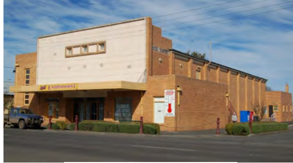
Koroit Memorial Hall (VHR H2222)
