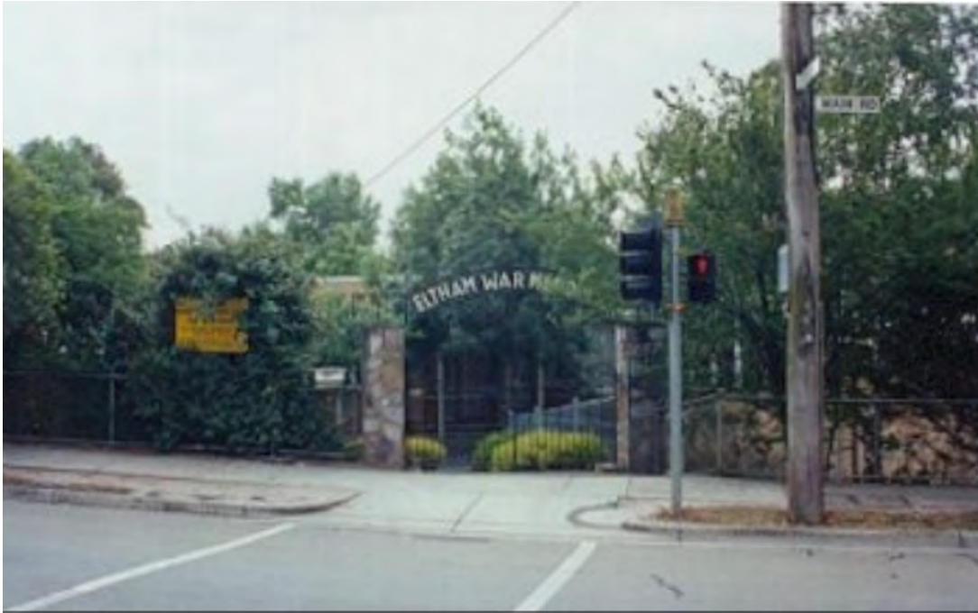
c1990s, Main Road frontage. Source: Victorian War Heritage Inventory.
