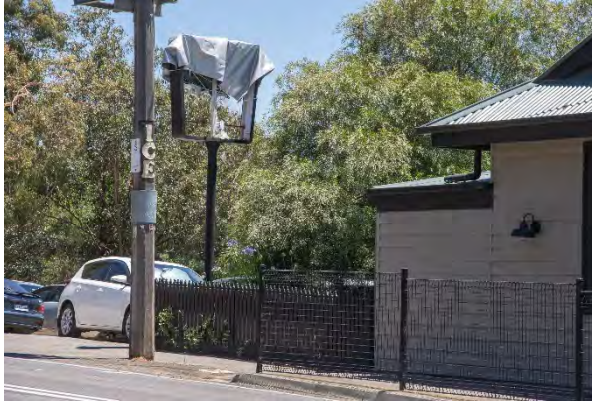
Figure 17. Southwest corner of the building and unused sign. (Source: Context 2020)
