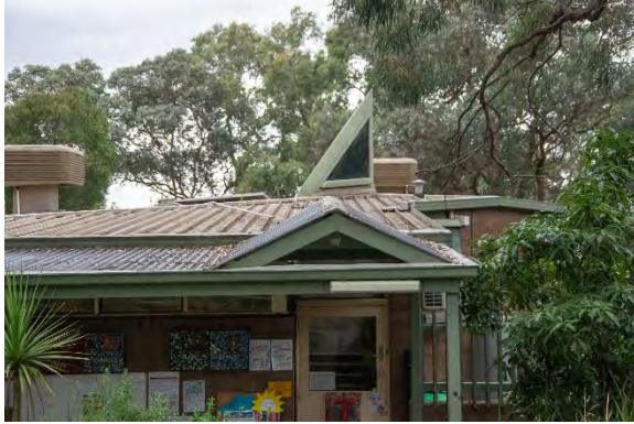
Figure 14. Small gable at main preschool entrance set above a skillion roofed verandah extension clad in corrugated iron. (Source: Context 2020)
