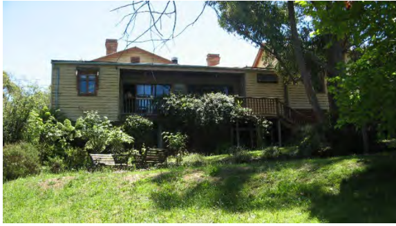
Southernwood, 250 Bolton Street, Eltham (VHR 2235, HO13). (Source: VHD)
