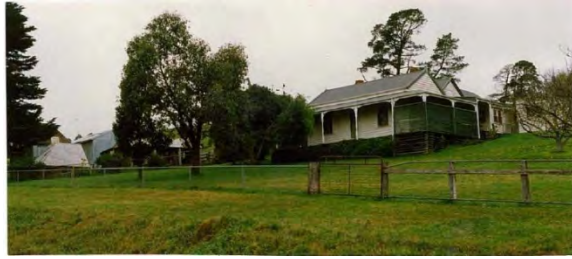
Weatherboard farm house and outbuildings, 760 Hurstbridge-Arthurs Creek Road, Arthurs Creek (HO89). (Source: VHD)
