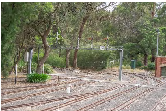
Figure 15. A portion of track. (Source: Context 2020)
