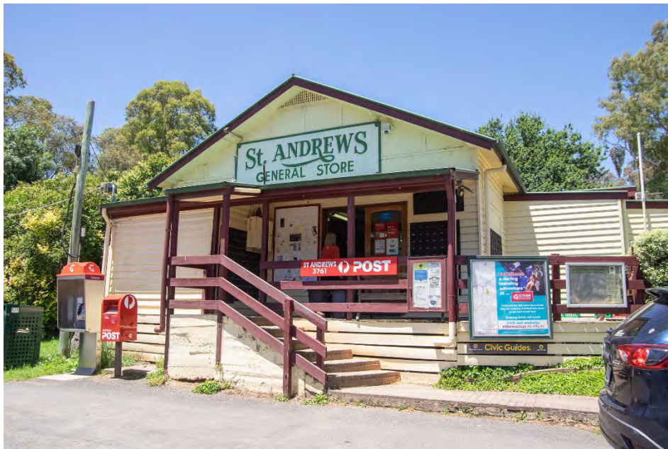
Figure 1. St Andrews General Store and House. (Source: Context 2020)
