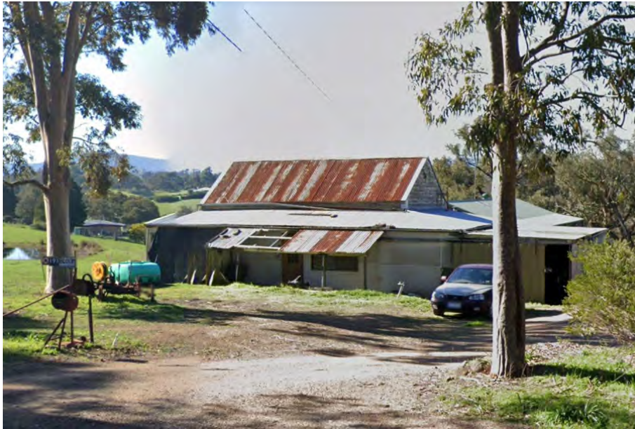
Figure 21. The primary (south) elevation of 191 Cherry Tree Road, with an attached garage, replaced window and door joineries and extended verandah. (Source: Google 2019)
