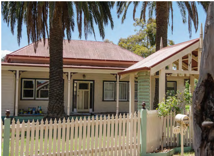
Figure 1. ‘Wendouree’ at 125 Cherry Tree Road, Hurstbridge. (Source: Context 2020)
