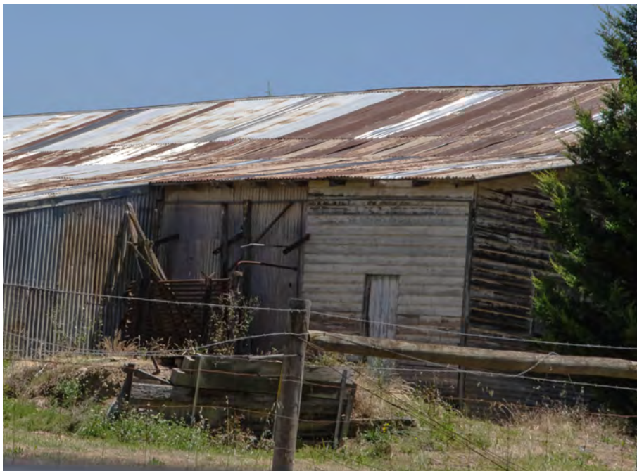
Figure 2. 180 Cherry Tree Road, Hurstbridge. Detail of the cool store showing the early timber section. (Source: Context 2020)
