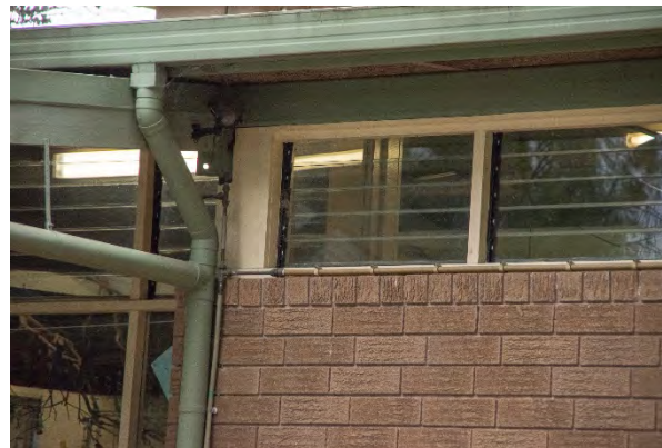
Figure 17. Detail of the glass louvred clerestory windows on the eastern side of the preschool (Source: Context 2020)
