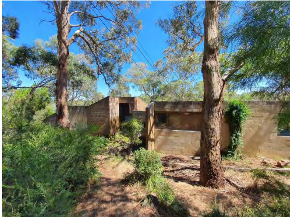
Figure 4. Entry to the house is via a narrow earth path leading past a series of interlocking geometric forms. (Source: Context 2021)
