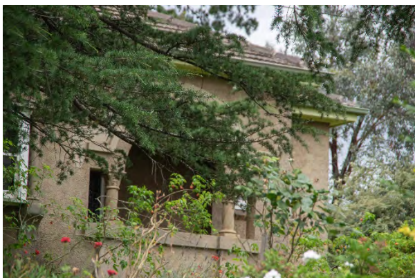
Figure 12. Porch arch with loose barley twist columns and smooth capped balustrade. (Source: Context 2020)
