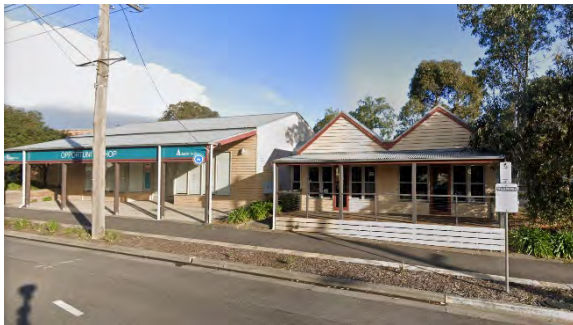
Former Milthorpe Store, 42-44 Main-Hurstbridge Road, Diamond Creek (HO259). (Source: Google 2019)
