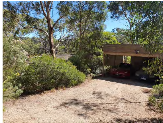
Figure 7. The carport to the front of the house and is enclosed on two sides with concrete block walls. The deep fascia across the front is clad in horizontal timber weatherboards (Source: Context 2021)
