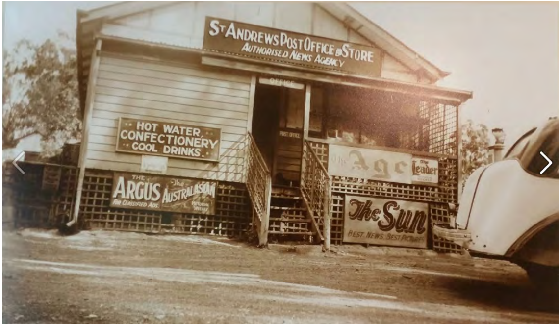
Figure 3. St Andrews Post Office and Store, c1930s. (Source: Facebook 2021)
