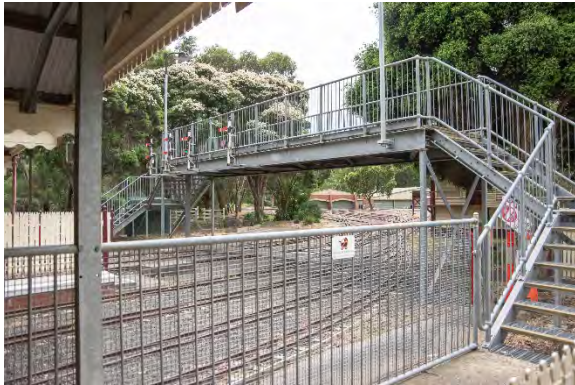
Figure 17. Steel-framed pedestrian bridge. (Source: Context 2020)
