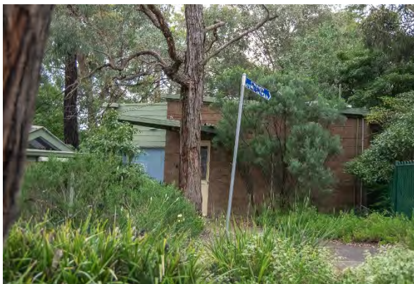
Figure 12. View of the infant welfare pavilion entrance from the carpark. (Source: Context 2020)
