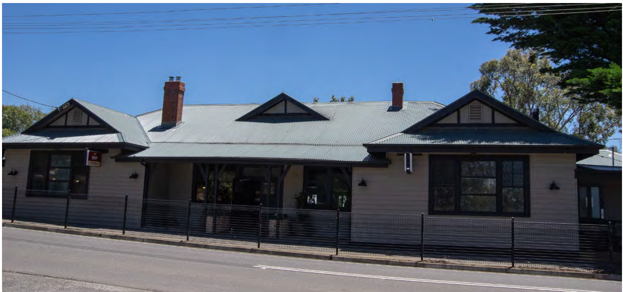
Figure 12. The primary elevation to St Andrews-Kangaroo Ground Road. (Source: Context 2020)
