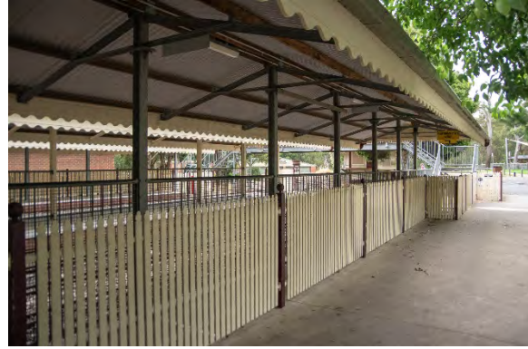
Figure 11. Picket fence and station canopy. (Source: Context 2020)
