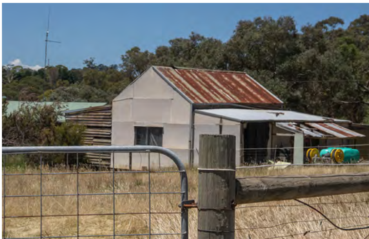
Figure 22. 191 Cherry Tree Road clad in painted sheets on the primary (south) and side (west) elevations. The window on the west elevation shown here and the verandah to the front of the house are later additions. (Source: Context 2020)
