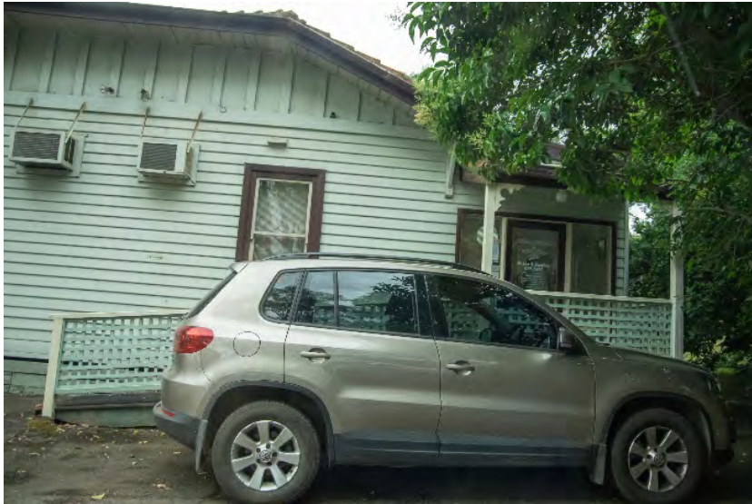
Figure 10. Secondary elevation showing weatherboard cladding with vertical batten detailing to the jerkinhead gable end, ramp and rear extension. (Source: Context 2020)
