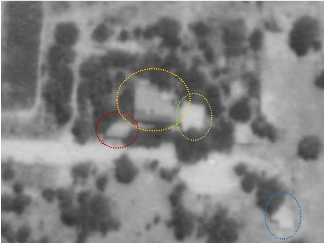
Figure 7. Close up of the subject site from 1951. The structures that existed on site by this time include: the 1948 study (outlined in red), the 1890s cottage (yellow), the c1948 rise addition with two rooms (green) and The Pottery built in 1950 (blue). (Source: 'MELBOURNE AND METROPOLITAN PROJECT NO.2' 1951 via LANDATA)
