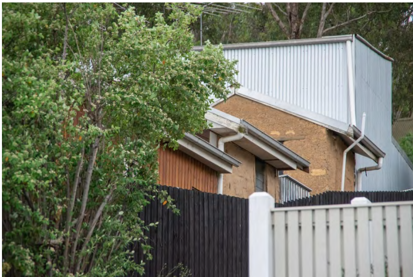
Figure 2. 42 Park West Road (front) and 1/44 Park West Road (rear), Eltham. (Source: Context 2020)
