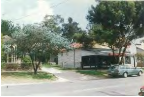
Weatherboard Shop, Corrugated Iron Building and Weatherboard House Behind, 960 Heidelberg-Kinglake Road, Hurstbridge (HO78). (Source: VHD)
