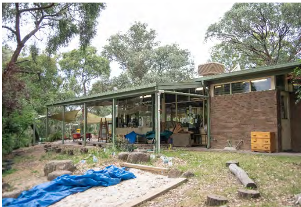
Figure 16. Sandpit and verandah on the eastern side of the building. (Source: Context 2020)
