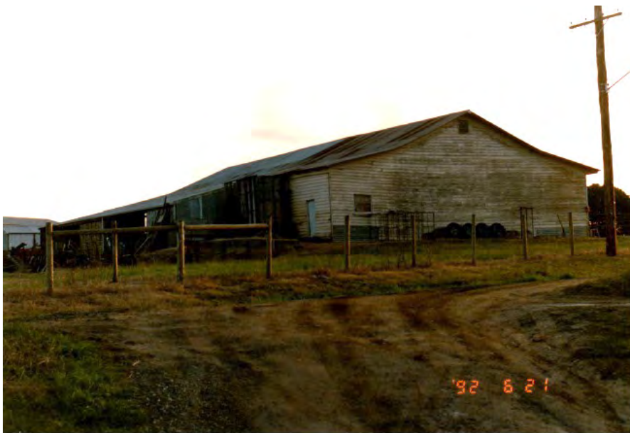
Figure 6. Cool shed at 180 Cherry Tree Road in 1992, viewed from the northwest (upper) and the northeast (lower). (Source: VHD)
