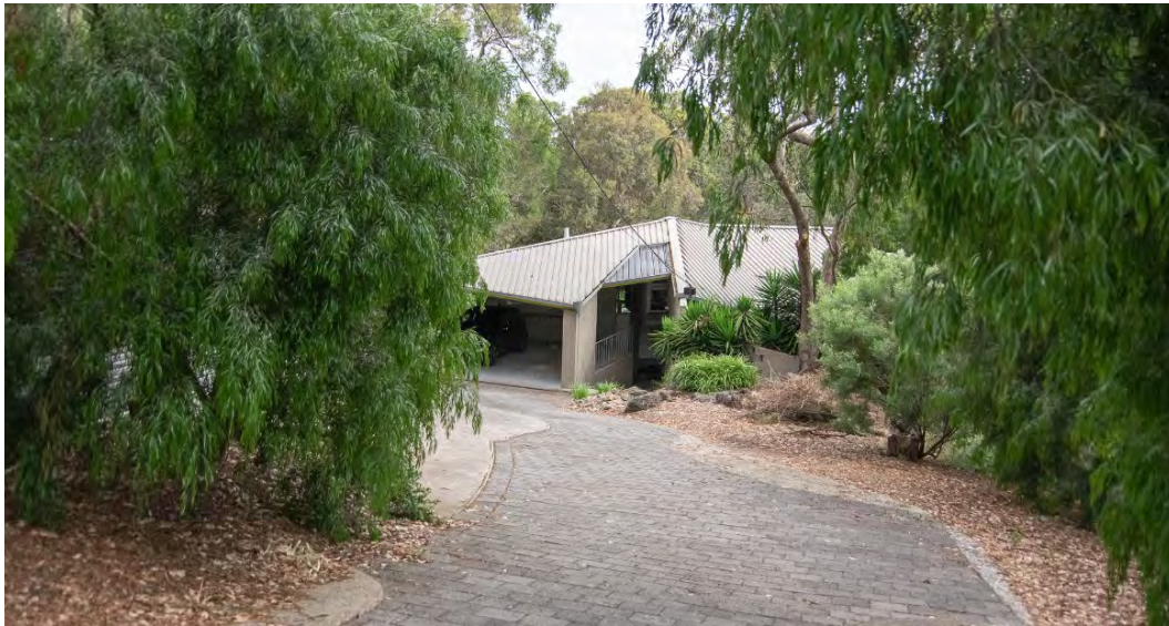
Figure 1. View of 144 Progress Road, Eltham North, from the street. (Source: Context 2020)
