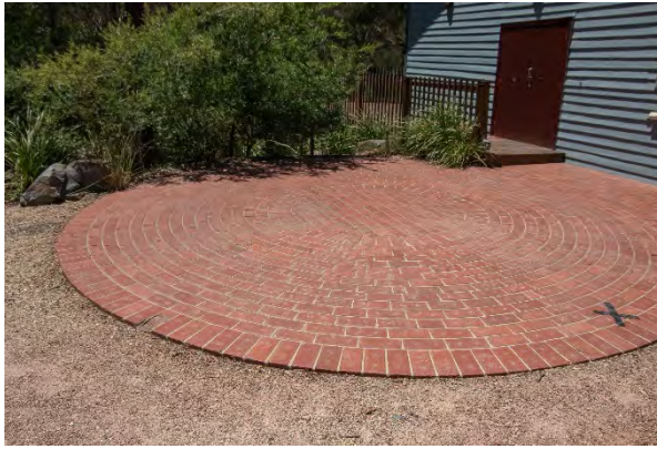
Figure 12. Red brick paving circle at the northern end of the building (Source: Context 2020)
