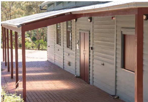
Figure 10. Corrugated iron verandah supported by timber posts over red brick paving. (Source: Context 2020)
