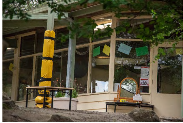
Figure 19. Window wall at the southern corner of the southern façade. (Source: Context 2020)
