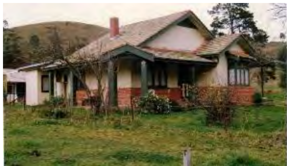
25 Cottles Bridge-Strathewen Road, Cottles Bridge (HO190). (Source: VHD)
