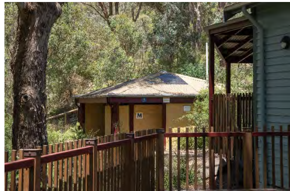
Figure 15. The toilet block viewed from the verandah to the rear of the building. (Source: Context 2020)
