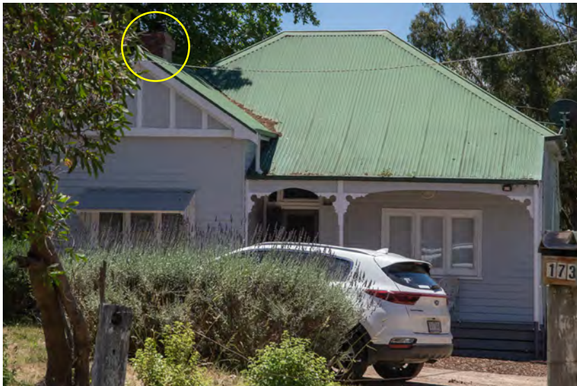
Figure 18. 173 Cherry Tree Road, with a projecting gabled bay with half-timbering detailing. Note the face brick chimney behind the projecting bay (outlined in yellow). (Source: Context 2020)
