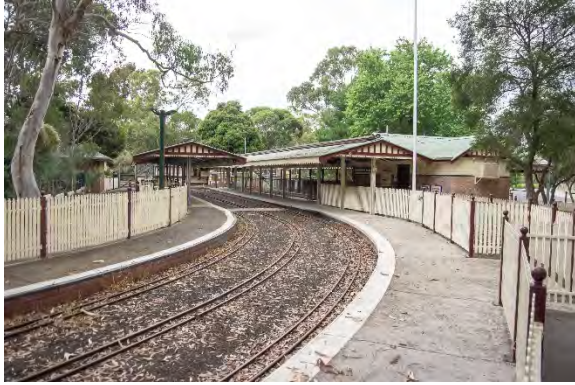
Figure 10. Main station platform. (Source: Context 2020)
