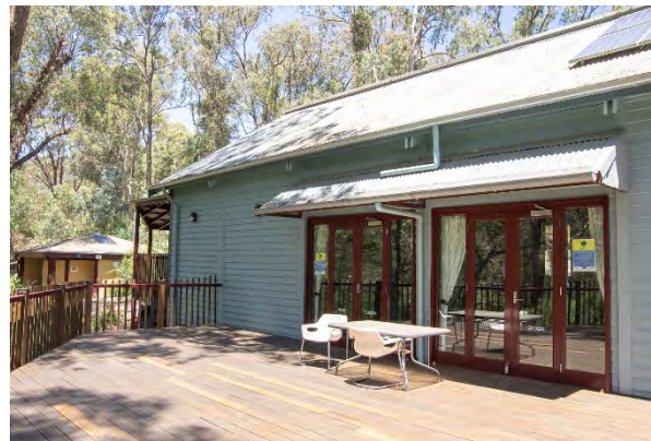
Figure 11. timber decking and row of glazed doors with shallow corrugated awning. (Source: Context 2020)
