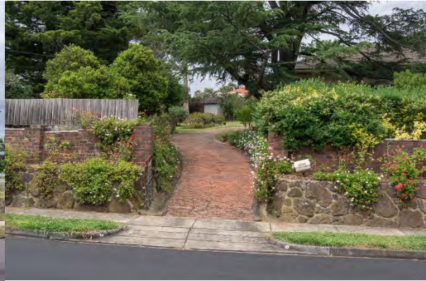
Figure 11. Red brick driveway from Batman Road with timber topped brick fence to the left. (Source: Context 2020)
