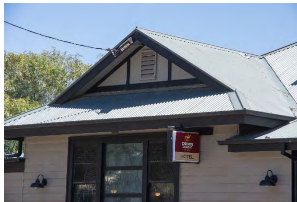
Figure 16. Projecting gable-ended bay. (Source: Context 2020)
