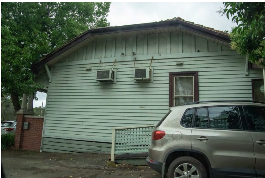
Figure 2. Side (south) elevation of 856 Main Road, Eltham, from the carpark. (Source: Context December 2020)
