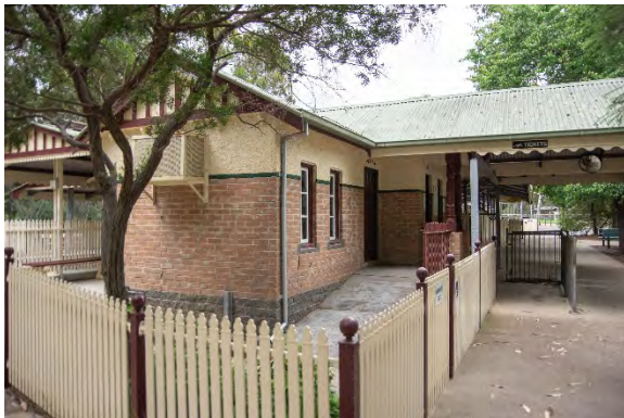
Figure 6. Station building with scalloped fascia. (Context 2020)
