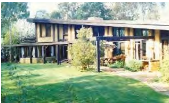
Pittard Residence, 430 Mount Pleasant Road, Research (HO139). (Source: VHD)
