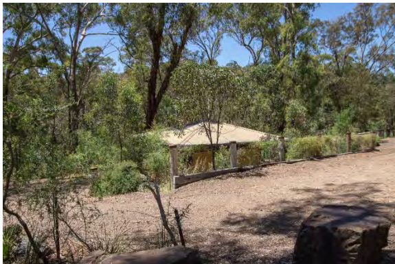
Figure 14. The toilet block sitting below a retaining wall. (Source: Context 2020)
