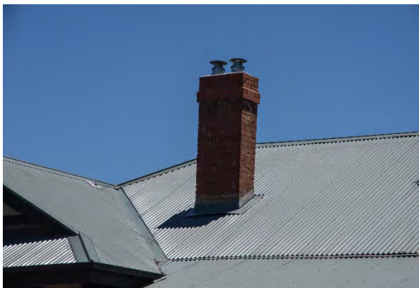
Figure 15. Brick chimney extending through the roof plane. (Source: Context 2020)
