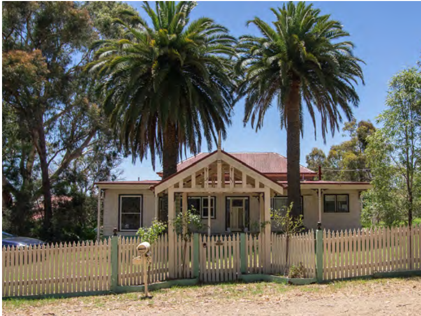
Figure 16. 'Wendouree' at 125 Cherry Tree Road, viewed from the south. The timber front fence and covered gateway is a later addition. (Source: Context 2020)
