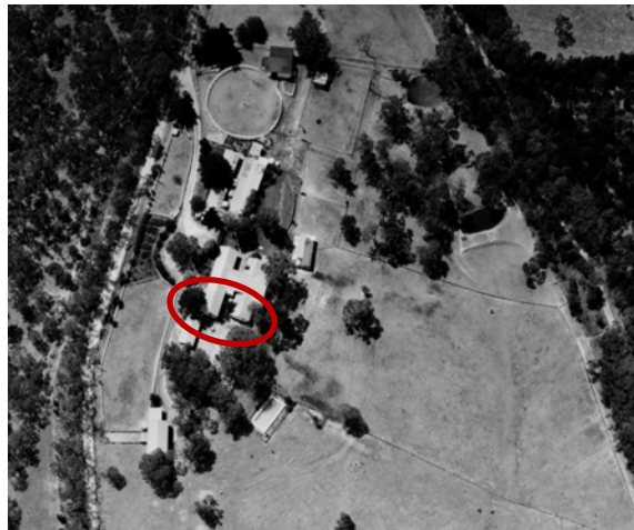
Extract of a 1978 aerial, showing the 1976 extension to the south of the existing dwelling (in red outline). (Source: Central Plan Office)
