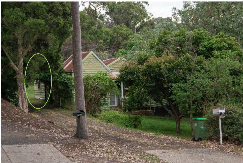
Figure 8. 23 Glen Park Road, Eltham North, viewed from the southwest. Note the rear extension clad in wider weatherboards (outlined in green). (Source: Context 2020)
