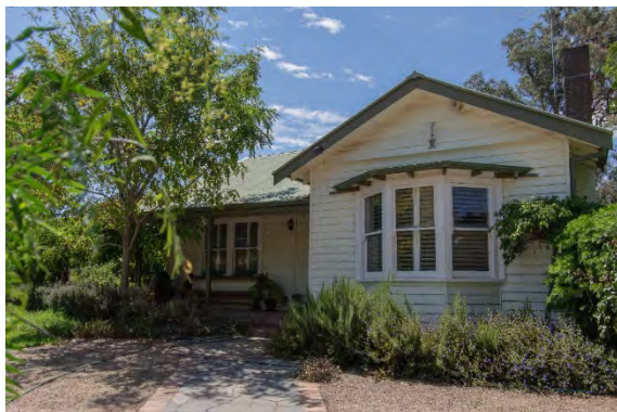
200 Ryans Road, Eltham North (recommended as Individually Significant in this study). (Source: Context 2021)
