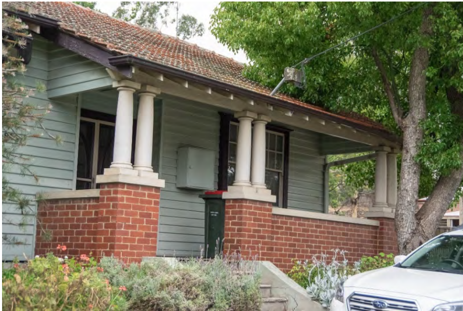
Figure 1. Primary (west) elevation of 856 Main Road, Eltham, with projecting verandah. (Source: Context December 2020)
