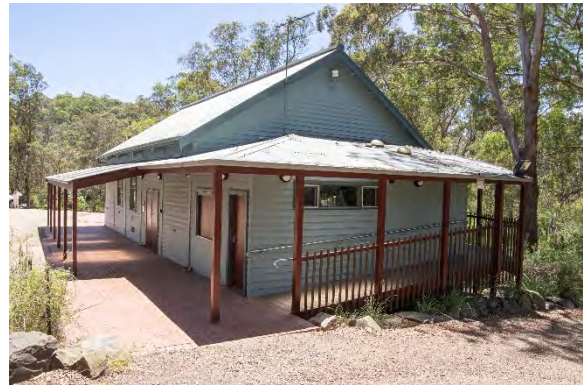
Figure 9. Rear of the hall, including ramp and kitchen addition. (Source: Context 2020)
