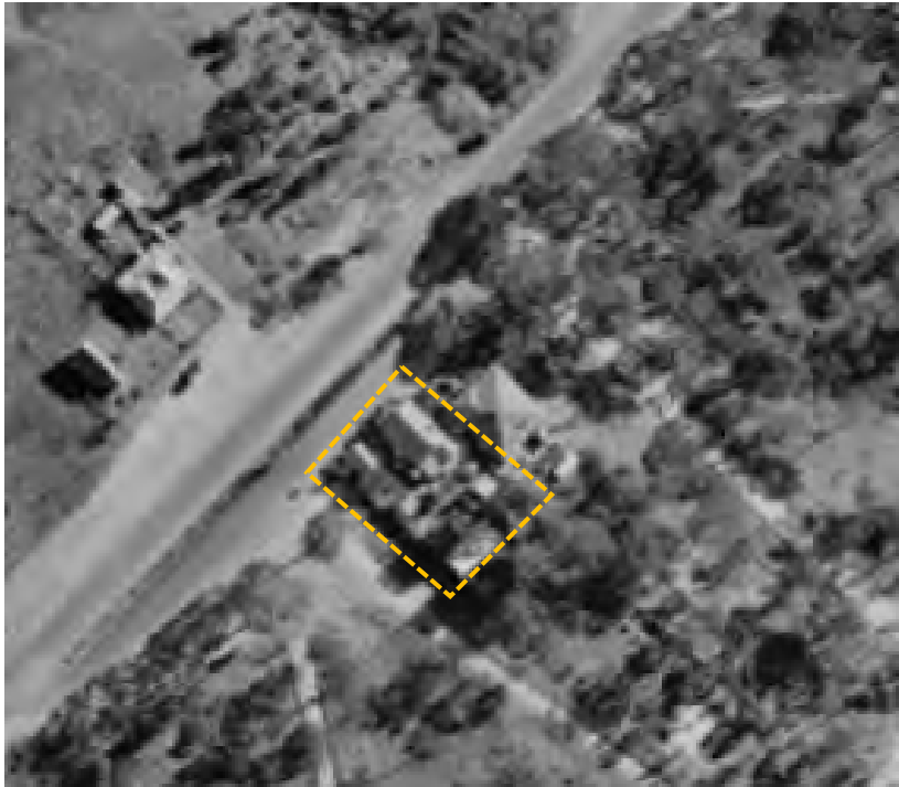
Figure 5. The subject site in 1968. The roof of the rear additions appear different from that of the mudbrick extension. The buildings on the subject site are approximately outlined in orange. (Source: CPO, 'MELBOURNE 1968 PROJECT', via Landata)
