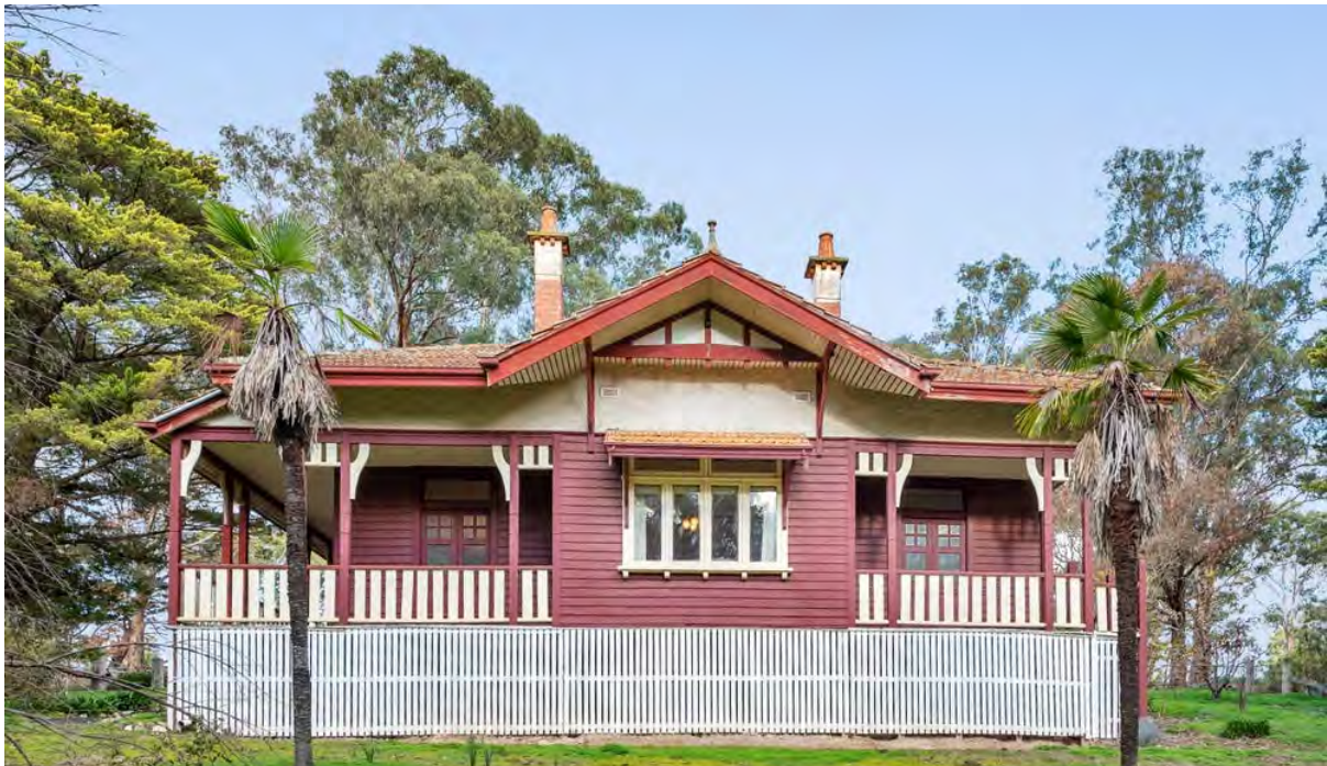
Figure 6. The northwest elevation. Note the projecting gabled bay, roughcast render panel beneath the eaves line, window awning and decorative timber fretwork to the verandah. (Source: realestate.com)
