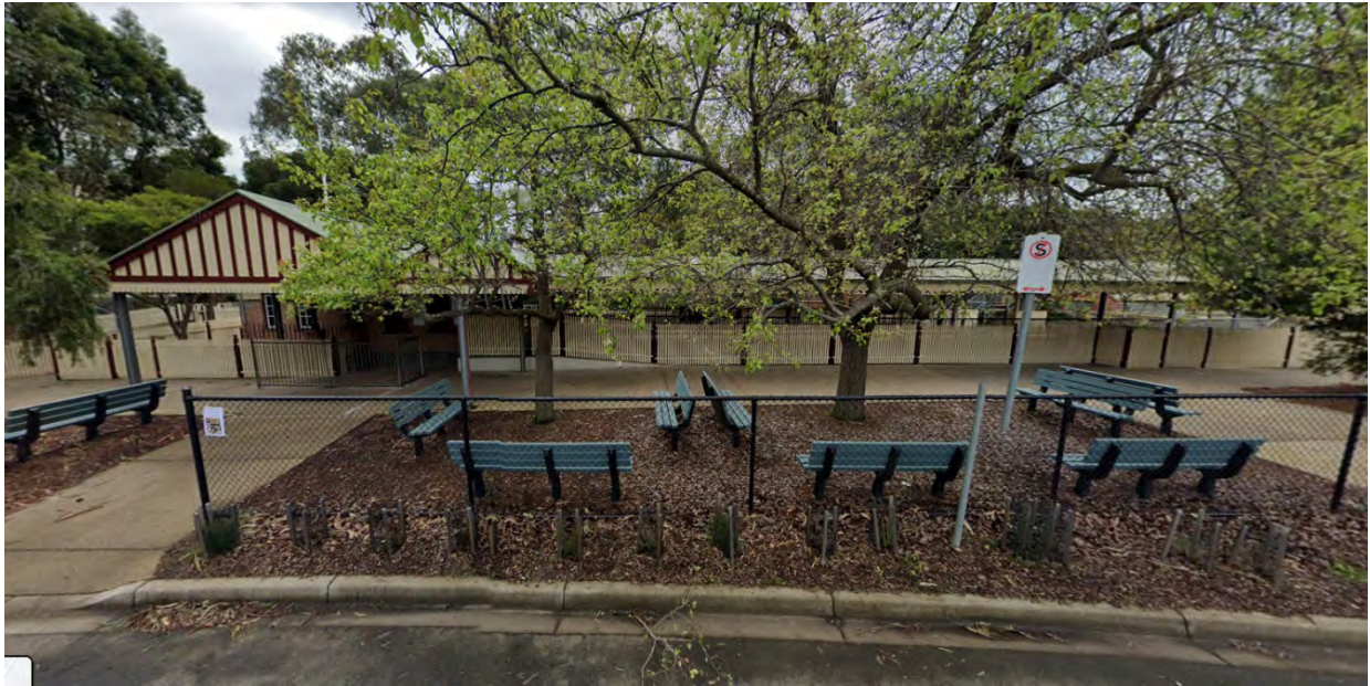
Figure 4. Primary entrance to the Main Station building (southwest elevation). (Source: Google Streetview 2019)
