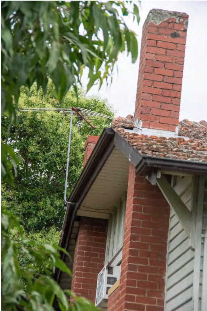
Figure 8. Two red brick chimneys on the northern elevation penetrate the jerkinhead gable. (Source: Context 2020)
