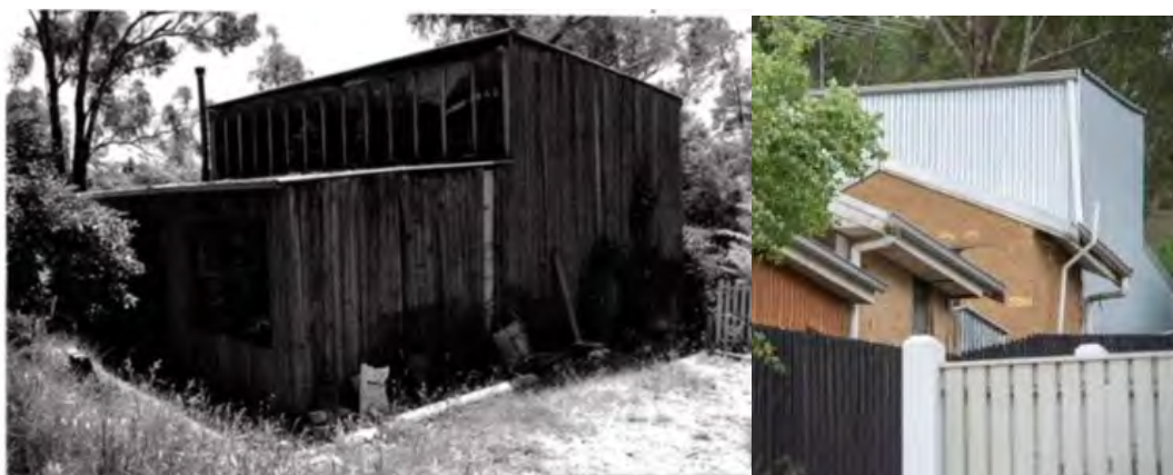
Figure 5. A c1992 image of the studio on the left, showing its original timber cladding. To the right is a current view of the studio, with new corrugated iron cladding. The small mudbrick room is visible in this image. (Source: Bick 1992; Context 2021)
