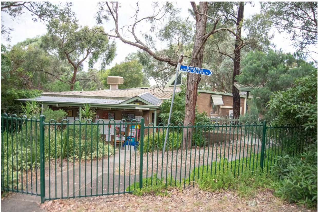
Figure 9. The entrance to the Preschool from the carpark showing the pathways to both pavilions and concrete stairs behind the aluminium fence. (Source: Context 2020)
