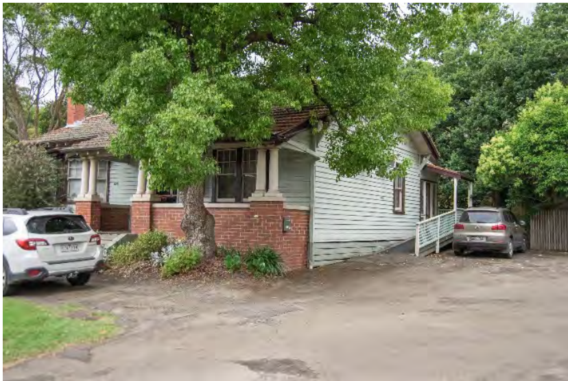
Figure 9. View of 856 Main Road from the southwestern corner. (Source: Context 2020)
