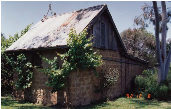
Peter Garner mudbrick studio and adjacent shed 62 Brougham street, Eltham (HO17). (Source: VHD)
