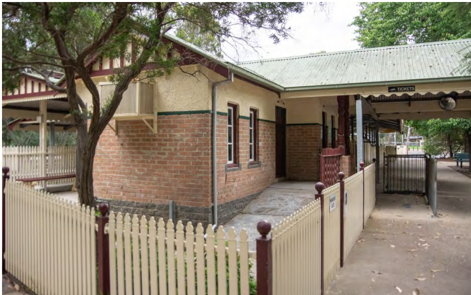
Figure 2. Main railway station building of the Diamond Valley Miniature Railway. (Source: Context 2020)
