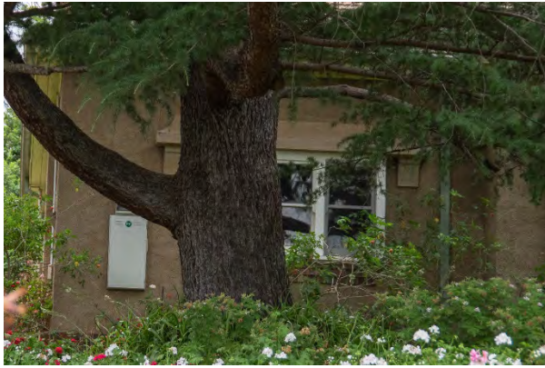
Figure 14. Second tier window detailing, with stepped brick sills and broad smooth rendered lintel supported by corbels. (Source: Context 2020)
