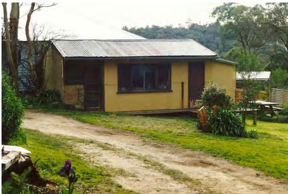
Alan Marshall Bungalow, 13 Park West Road, Eltham (HO147). (Source: VHD)
