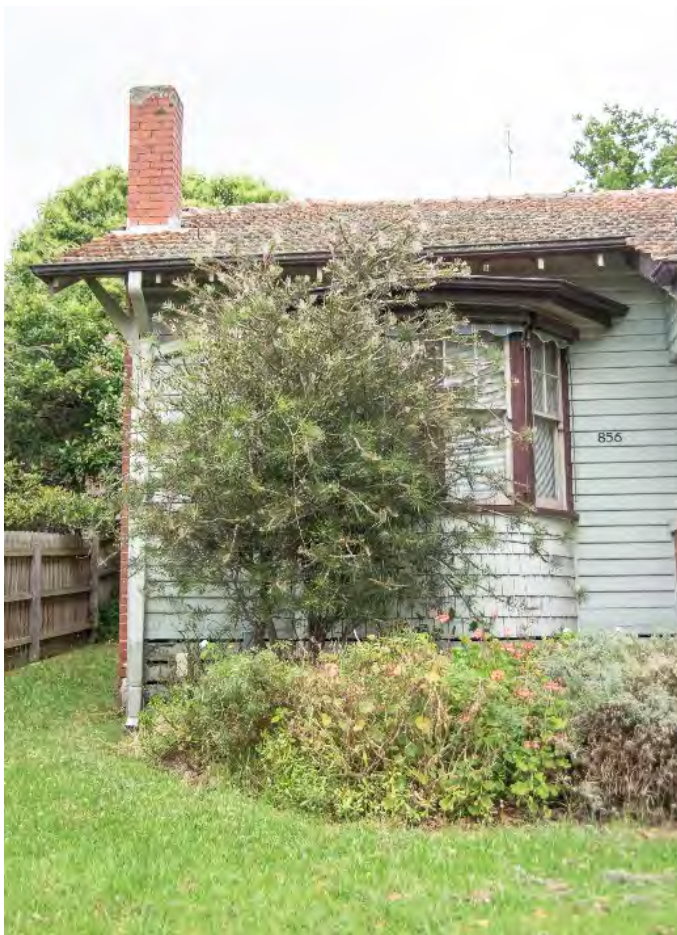
Figure 7. Bow window with canopy on the northern side of the main elevation with shingles. (Source: Context 2020)
