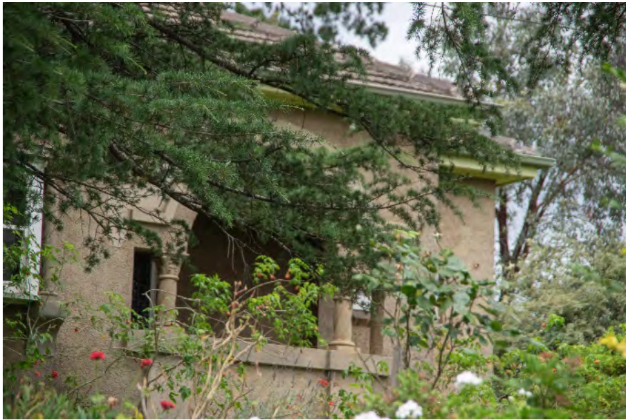
Figure 1. 2 Batman Road, Eltham, detail of the primary elevation with Mediterranean detailing. (Source: Context 2020)
