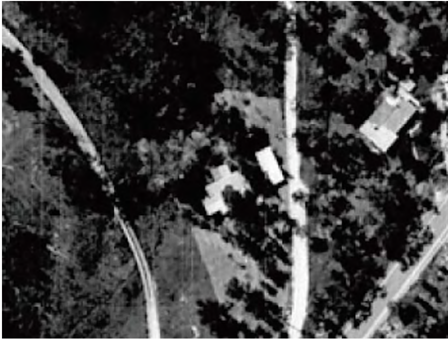
Figure 5. Aerial view of the Janeba House in 1963. (Source: CPO, 'Melbourne 1963', 1963 via Landata)
