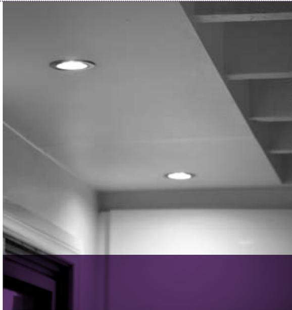
**Test your LEDs – sometimes compatibility issues occur between the LED lamp and transformer, so purchase one lamp first and test it before buying replacements for all lights.**
