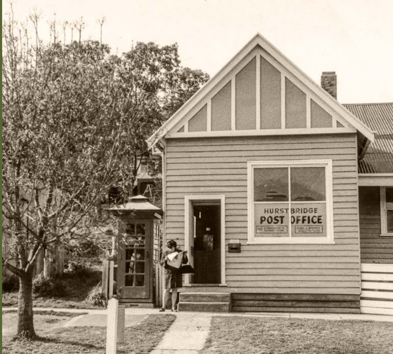
The Hurstbridge Post Office was originally the office of the Evelyn Observer newspaper when the paper relocated from Kangaroo Ground.
