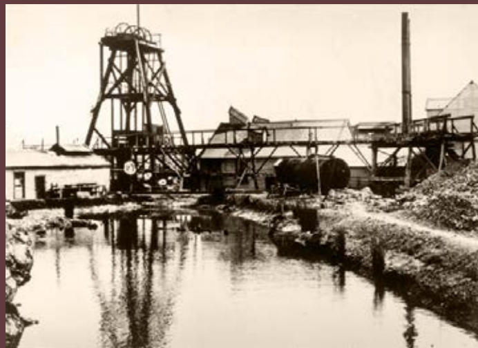
Diamond Creek Mine with single boiler, 1890
