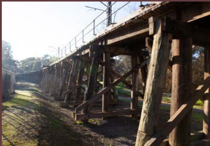
Eltham Trestle Bridge, 1981 The Shire of Eltham Office in background
