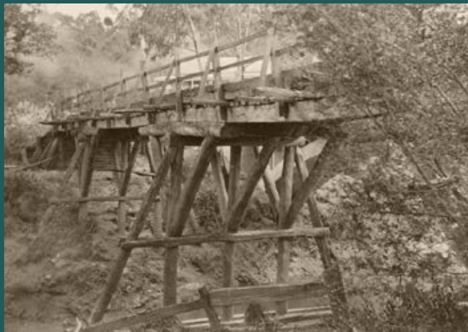
Opening of the Monash Bridge, 3 November 1917
