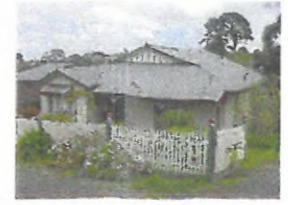
← 1 0 No. 36-38 Old Aqueduct Rd
