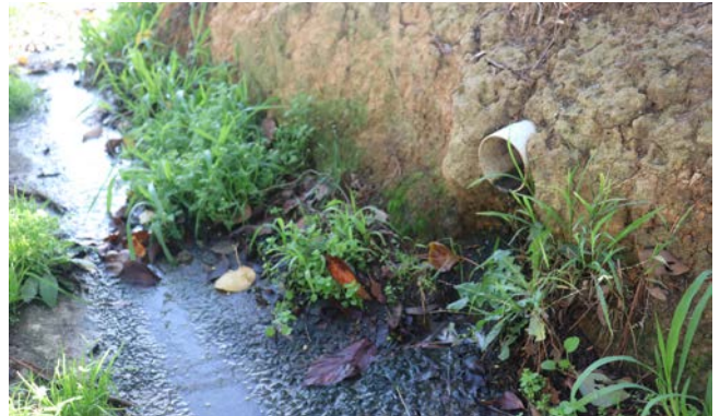
Figure 1: Greywater discharge to street culvert in Howell Road, Plenty
