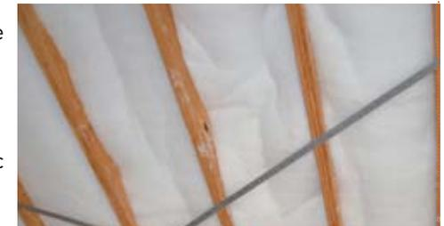
Bulk insulation works by trapping heat in the small air pockets throughout the product. If bulk insulation is compressed it will not work effectively, so a batt should fit snugly into the allocated space, but not be squashed in.
