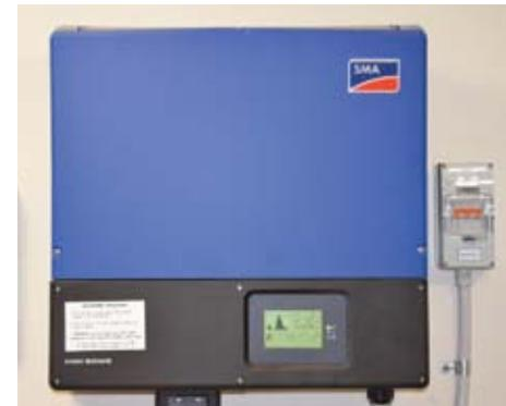
**The inverter must be sized appropriately for the system or slightly larger than the power output of the panels to allow for future expansion.**
