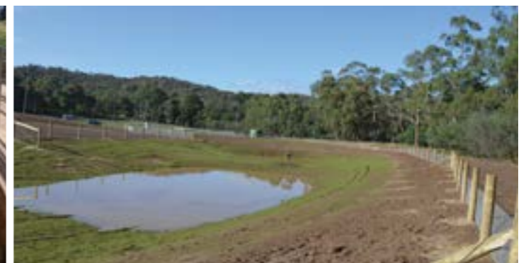
Hurstbridge Wetland post construction (July 2014)
