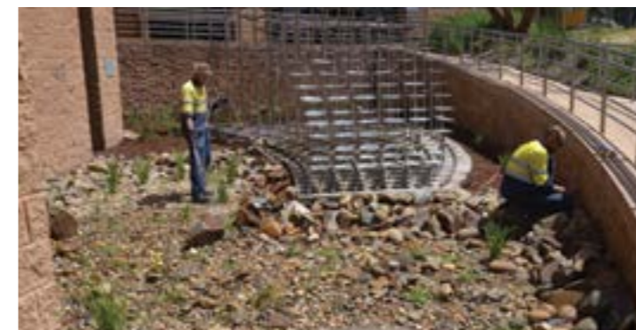
Shire Office Raingarden under construction (January 2015)
